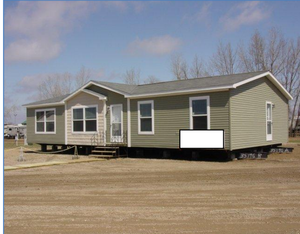
Mobile/Manufactured Home Skirting will be installed when the home is delivered to a permanent location.
