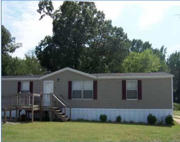
Mobile Home/Manufactured Home Skirting has been installed covering the chassis.
