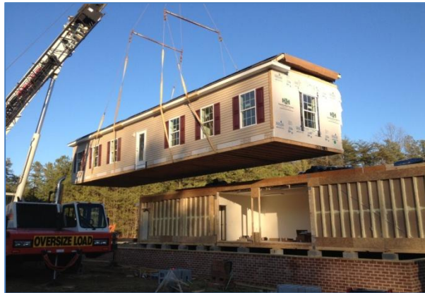
Modular Home (Under Construction) Individual modules delivered to the site and assembled on a permanent foundation
